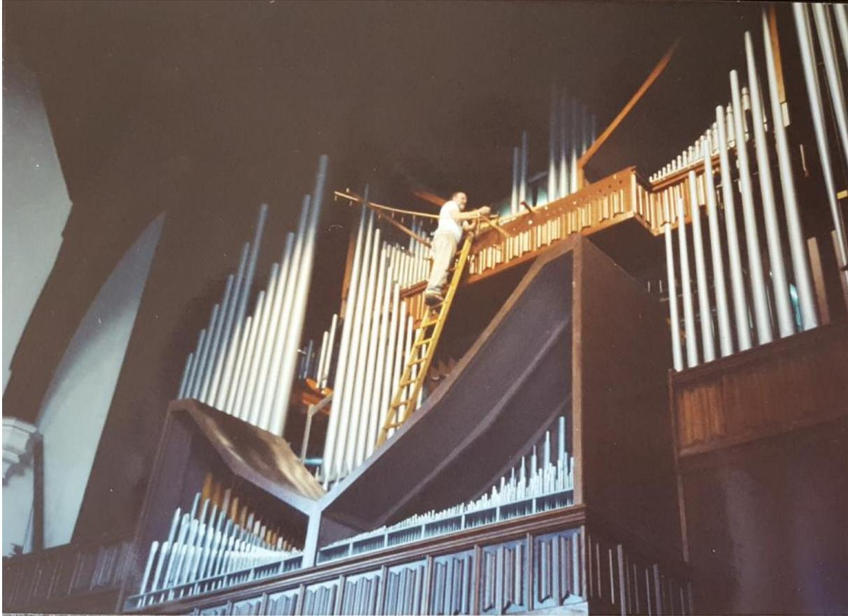
Figure 10. The *Trompette-en-Chamade* pipes being installed.
