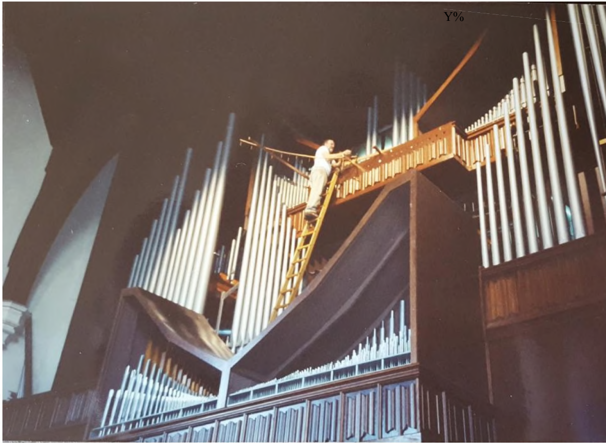
Figure 10. The Trompette-en-Chamade pipes being installed.
